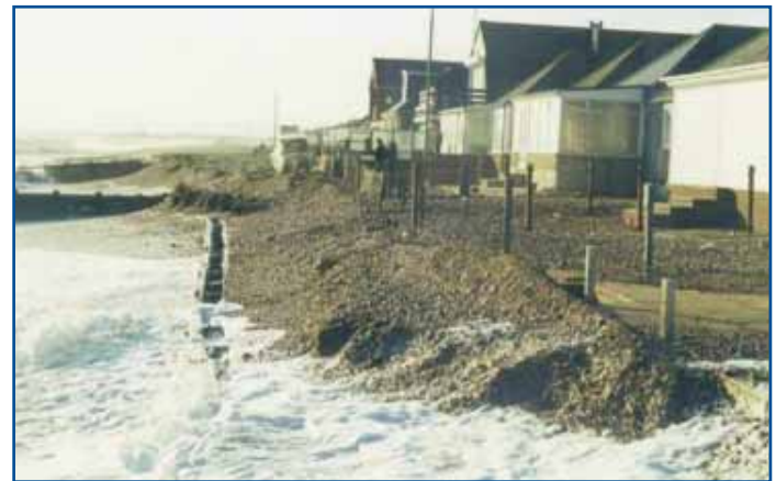
Figure 8 Typical erosion before improvement works (courtesy Pevensey Coastal Defence Ltd/Environment Agency)
