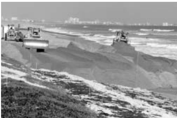
Beach nourishment and coastal restoration off the states of Florida
